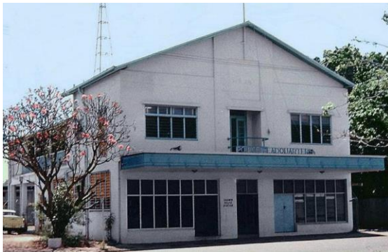
Figure 17 - Bennett Street Police Station and Police headquarters circa 1950s - the building was constructed as an arcade come residential building called the Mendis Building in 1941 but was eventually purchased by the Commonwealth Government.
