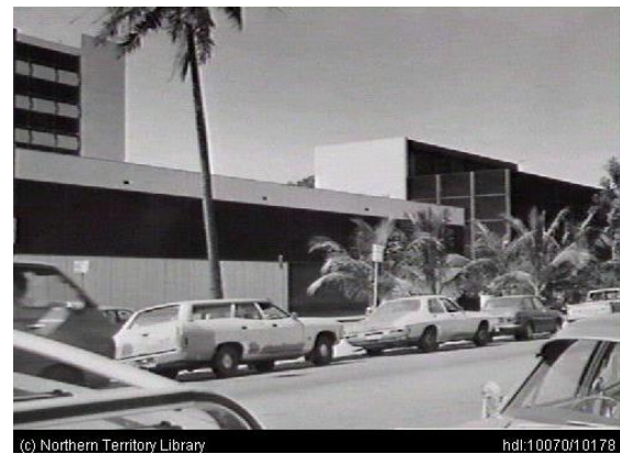
Figure 18 - the new 1970 Mitchell Street Police Station (photo taken in 1985)
