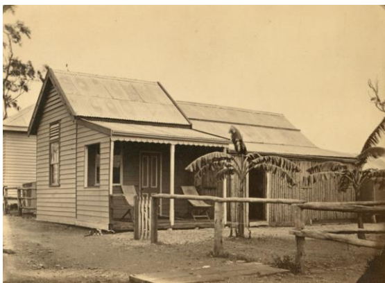
Figure 9 - Foelsche's Residence - next to the first Permanent Police Station
