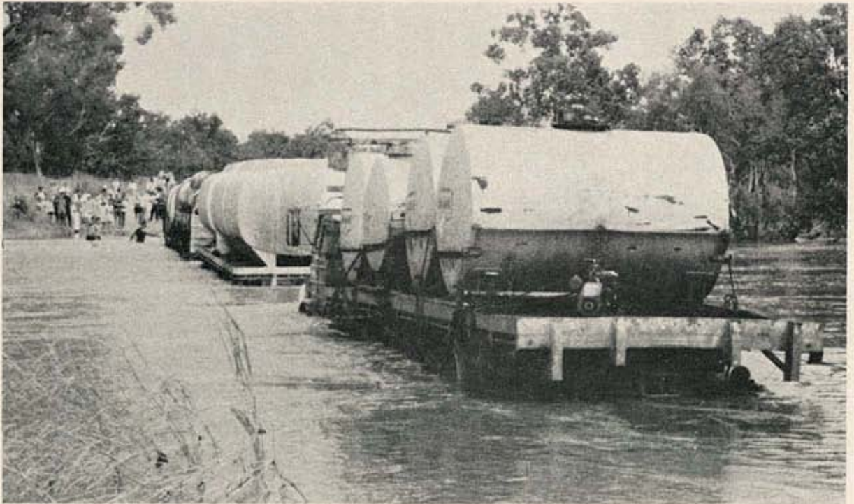
First across the Cullen River, after days of waiting vainly for the bridge surface to appear.
