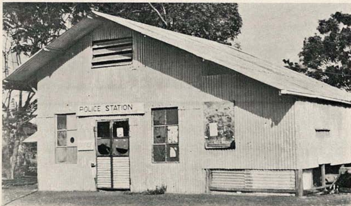
Policemen's Purgatory! — this angle-iron sweatbox was part of the "new" Police Station buildings referred to by Ted Morey. It was used as Police office and court room for nearly 40 years until the present brick replacement eventuated.
